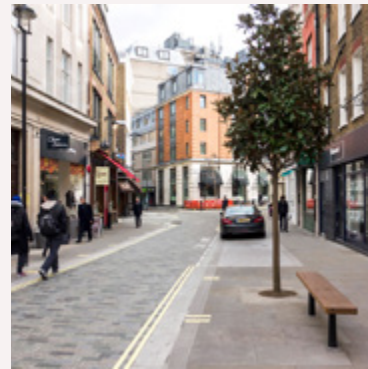
De-cluttered footway with raised loading pad, tree and seating on Marylebone Lane
