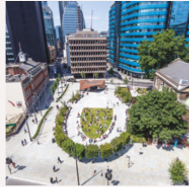
The removal of Aldgate Gyratory unlocked the possibility for a vibrant new public space (Aldgate Square).
