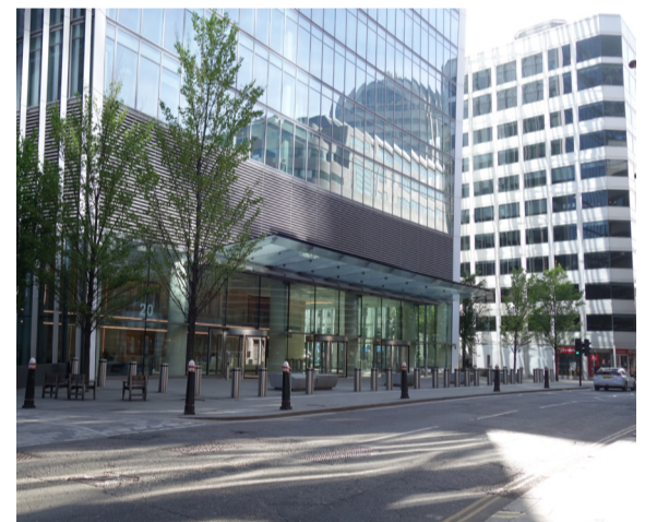
The frontage of 20 Fenchurch Street
