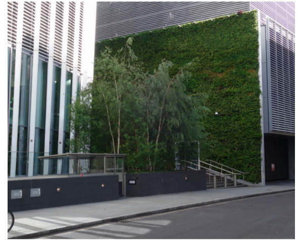
The green wall at the base of 20 Fenchurch Street
