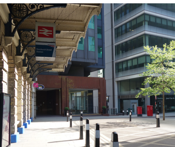
The station forecourt is level with a stepped route on its south side leading towards Tower Hill
