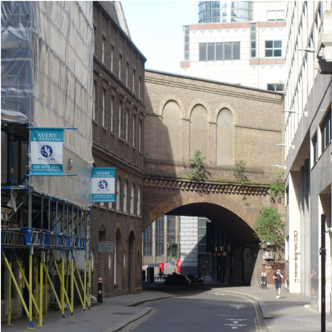
Crutched Friars is a dramatic street running underneath the station
