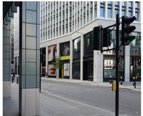
The double height base of 120 Fenchurch Street
